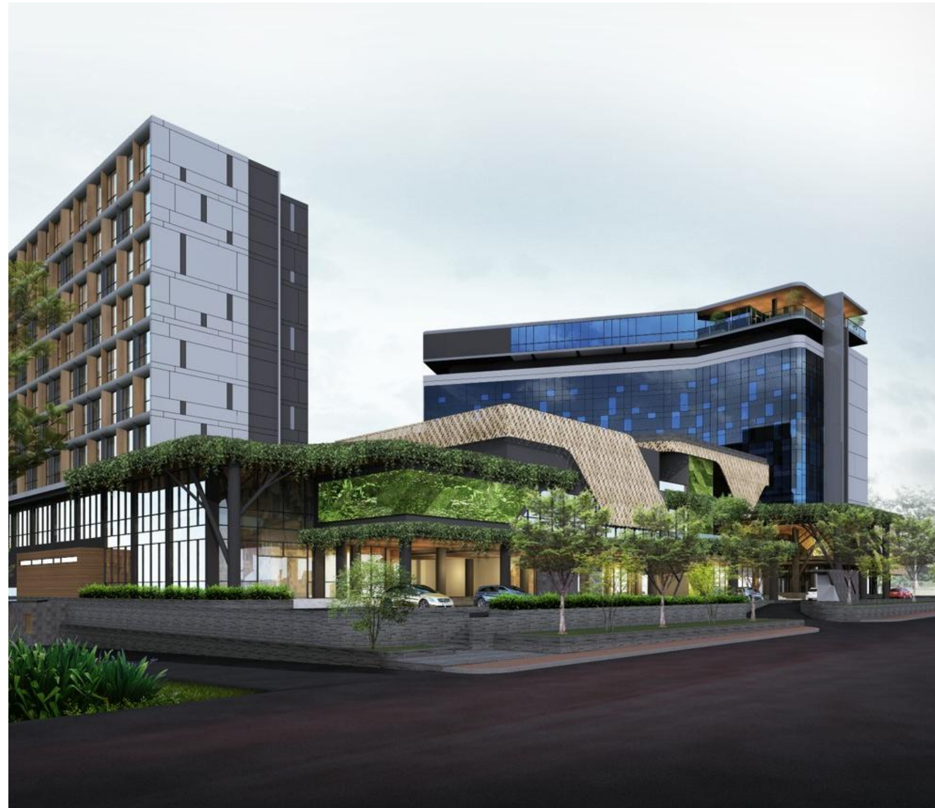
ibis Yogyakarta International Airport Kulonprogo, Indonesia | 224 rooms
